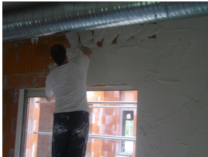
Figure 21. Plaster applied on interior wall.
