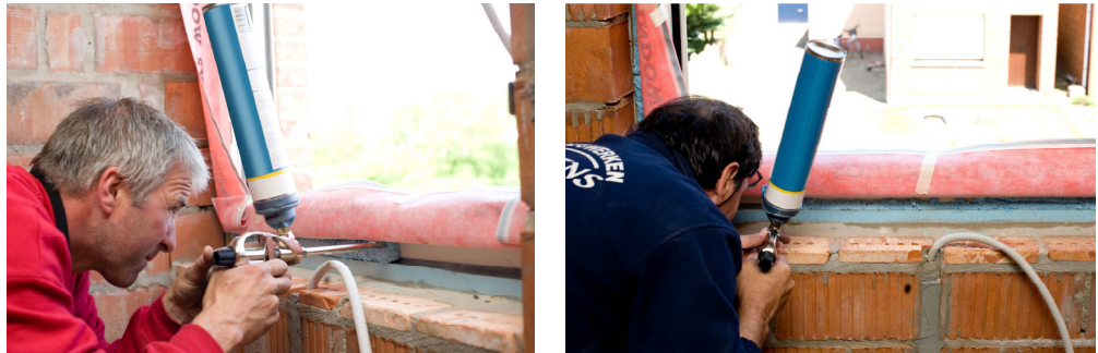
Figure 31. Application of elastic PU foam around a window. Courtesy Soudal.
