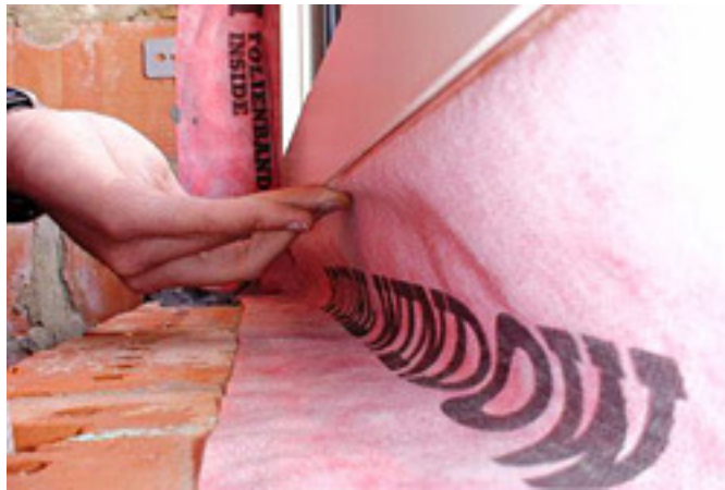
Figure 26. Application of a membrane around a window. Courtesy Soudal
