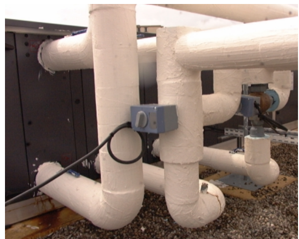
Figure 18 : View of heat pump (left) and three-way valve for heating power control (right)
