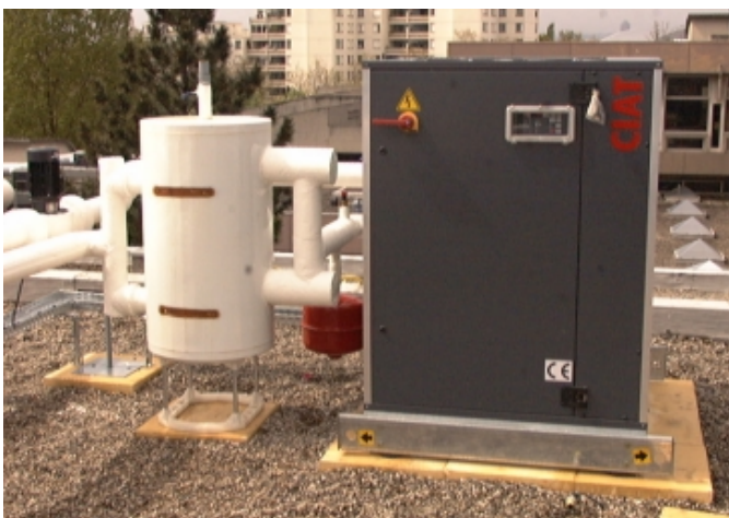
Figure 18 : View of heat pump (left) and three-way valve for heating power control (right)
