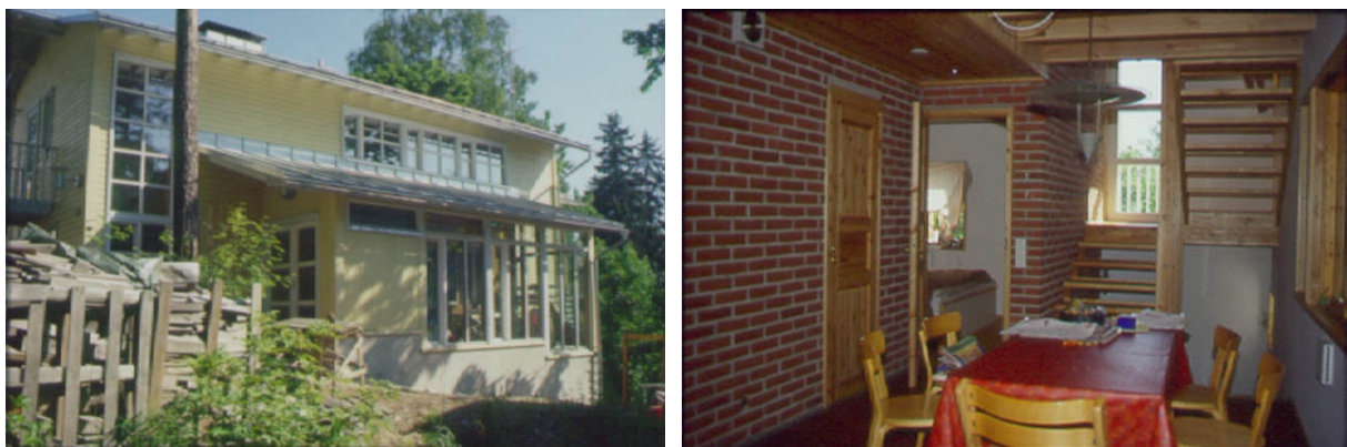
Figure 1. Pictures of the south facade and dining area of the test house (Riikka Kostiainen). The triple pane windows are concentrated on the south facade to take advantage of solar heat gains in the winter and to provide natural lighting to the house
