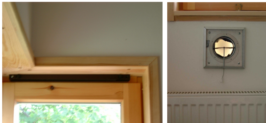
Figure 4. The house contains 13 supply air vents located in the upper window frame and 7 in the exterior wall above the hot water radiators. The occupants can control both types of supply vents. The supply vents above the radiators are seldom open, especially in the winter.
