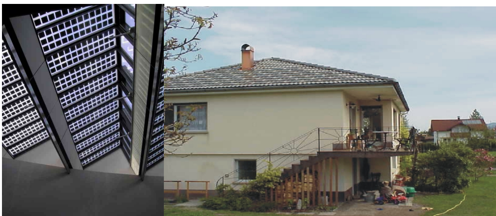
Figure 3 : Photos of Hip-Hip PV systems – Left : Sophisticated system design for the ISE building, Freiburg, Germany – Right : Solar tile application in Fussach, Austria
