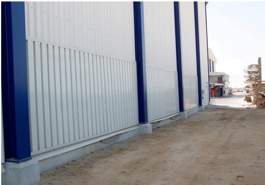
Installation of a typical sand tap louvres
