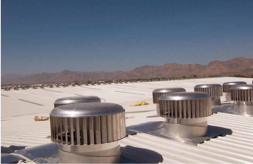
Installation of wind driven turbine ventilators
