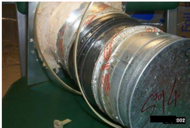
Figure 7. Failed plastic strapping on one of the flexible core to sheet metal collar specimens after four months of aging.
