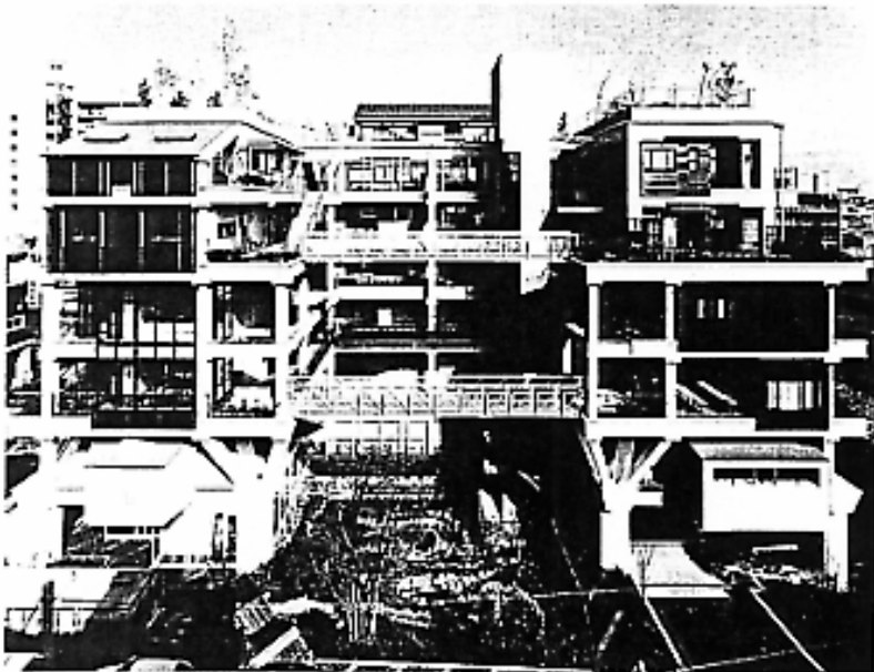
Photo-1 NEXT21 Total Floor Area 4577 M 2 Dwellings 18
