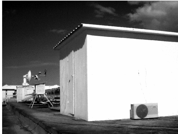
Fig 5 : Sight of the Test cell and the outdoor unit of the split-system.
