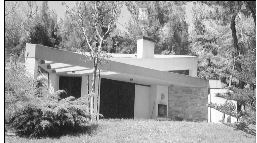
Figure 1: East facing elevation of the house.
