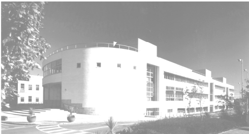
Figure 1: WIT Library Building (SW view).
