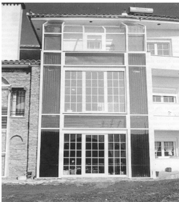
Figure 7: The solar-air collectors.
