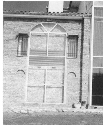
Figure 6: The Trombe wall.
