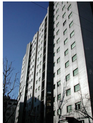
Figure 1: Photo of the building.
