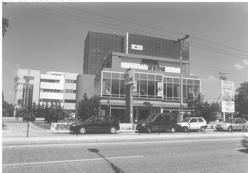
Figure 3: The existing building as seen from the avenue. (East elevation).
