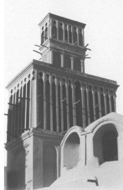
Figure 5: Wind tower in Abarghoo.
