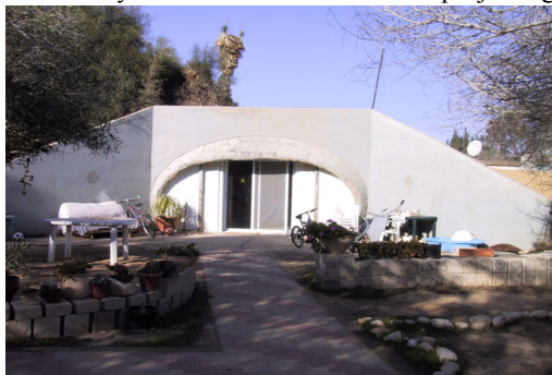
Figure 8: Earth Covered Building in Sde Boqer, Israel. South View.
