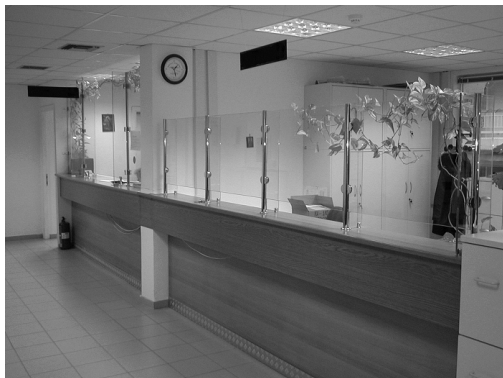
Figure 3: Views after retrofitting actions; 1 st case study (upper) and 2 nd case study (lower). Ventilation grids embedded in the suspended roofs for hybrid and mechanical ventilation.
