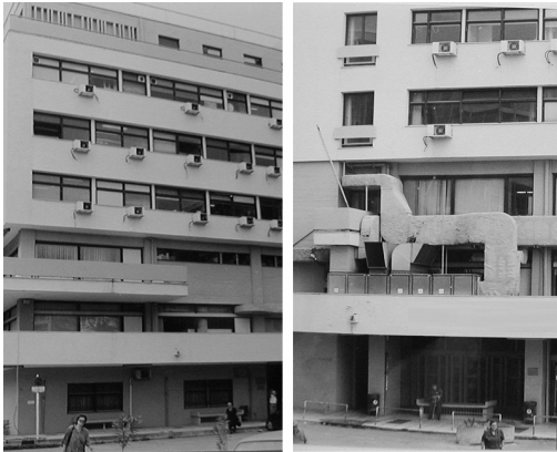
Figure 1: Views of the building of the first case study before retrofitting actions. Old split A/C units and windows (left) and old duct A/C systems (right) before the removal and their effect on the building's aesthetics.
