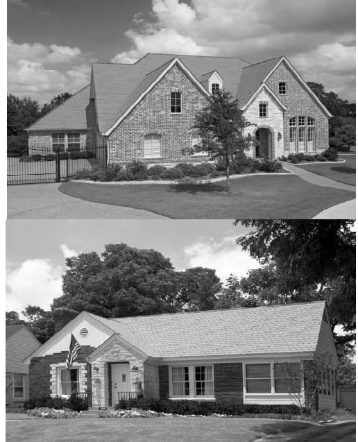
Figure 7: Test application of cool colored roofing shingles on two houses.
