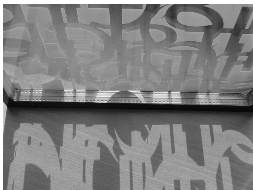
Figure 6: Double-glazed IMERA element with screen printing as sun protection and design feature.
