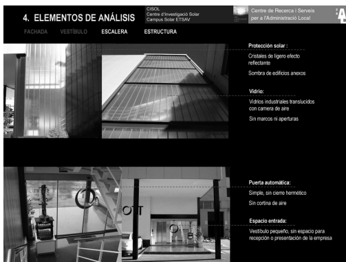
Figure 2: Building analysis and description of deficiencies.
