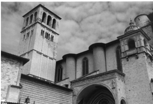
Figure 1: St. Francis Basilica Superior Church in Assisi (south oriented façade).
