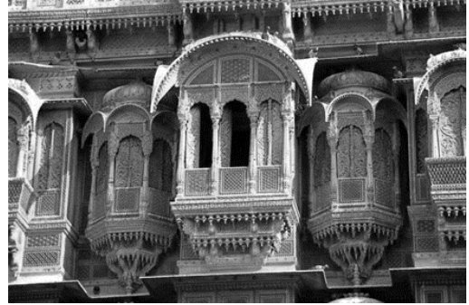
Figure 9: The haveli or balcony which is a wind inlet in the first floor of a merchant house in Rajasthan.
