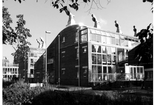
Figure 1: Beddington Zero Energy Development.
