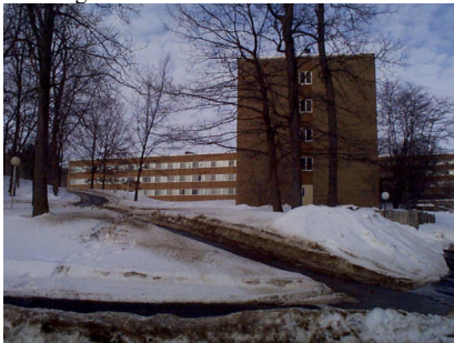
Figure 2: A picture of Bursley Hall Dormitory showing the south-west wing with its landscape.
