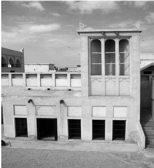
Figure 2: Great windcatcher in Bahrain where the hot humid climate requires that maximum air movement over the skin is achieved to stimulate evaporative cooling for summer comfort.
