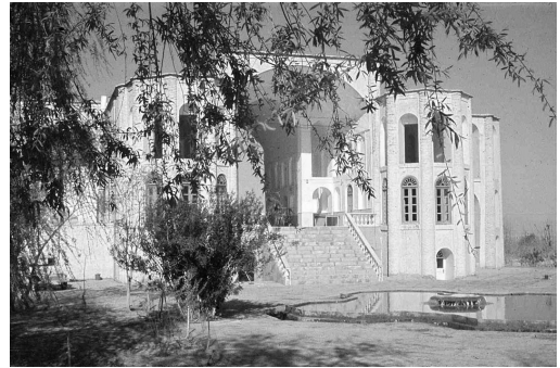
Figure 3: Pavillion of the Bagh-e Khan served by the windcatcher with chilled mountain air and water via a qanat canal.
