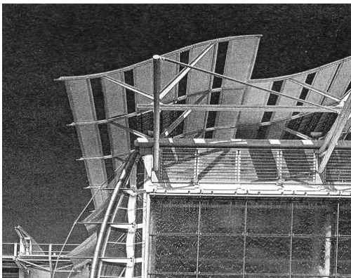
Figure 6: Solar "hats" on the roof, EXPO 1992.
