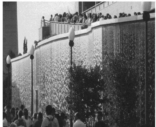
Figure 7: Water over glass façade.
