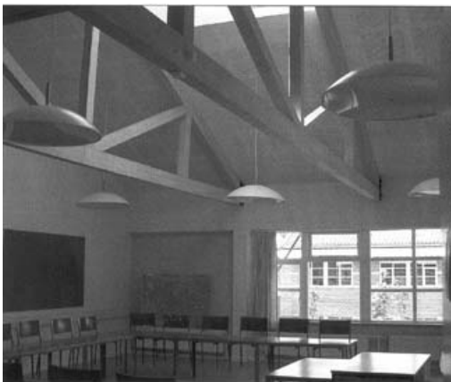
Figure 7: Photo showing the interior of a refurbished classroom.
