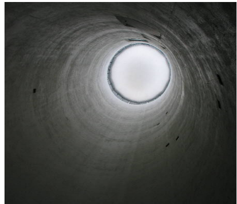
Figure 9: An interior view of the new air intake tower.
