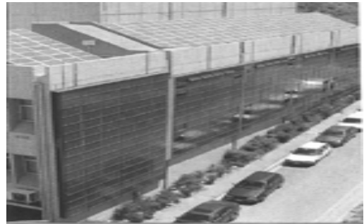
Figure 11: View of the Chem. Eng. building after retrofit.
