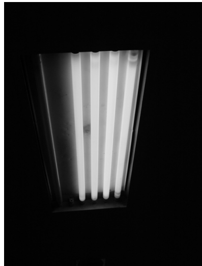
Figure 6: Typical luminaire with different CRI and CT.
