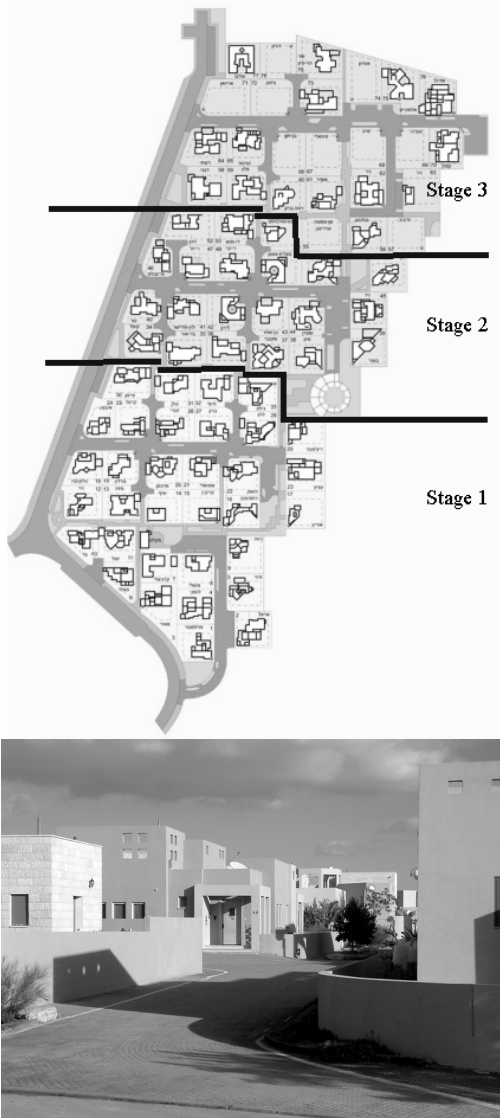
Figure 1: Top: Neve Zin solar neighborhood. Bottom: view of street demonstrating solar access on Dec.21 afternoon.
