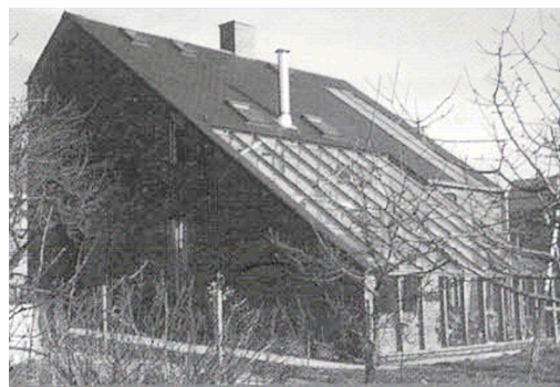
Figure 1: View on the house before renovation (design: ir. L. Vandaele).
