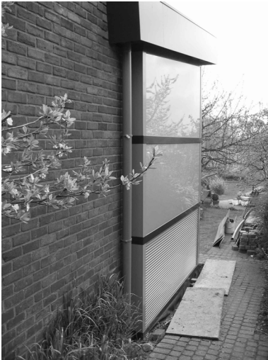
Figure 11: Louvre for night time ventilation at lower part of the West façade.
