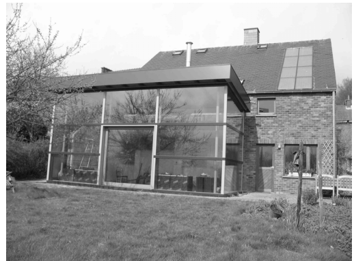
Figure 13: Status of the renovation works in April 2005, still without shading.
