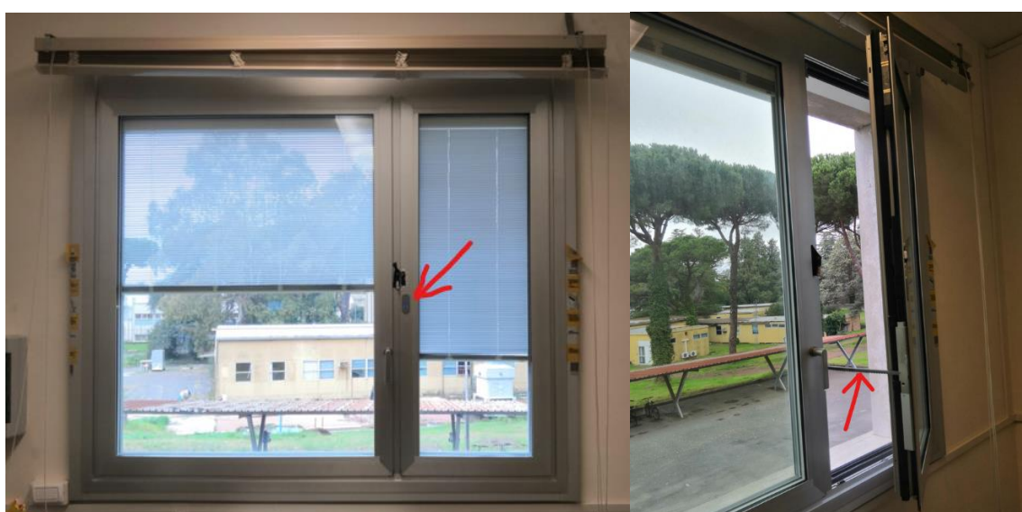
Figure 3: Front view of the new window, left, with the push-button indicated on the right sash; detail of the motorized chain to open/close the sash on the right.
