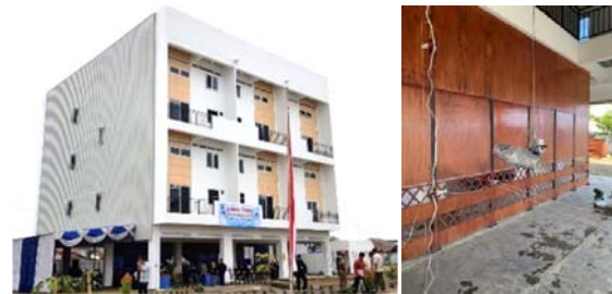
Fig. 2. Experimental house in Tegal, Indonesia.
