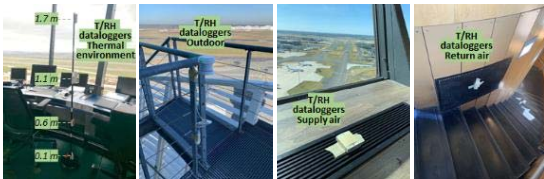
Figure 4. T/RH dataloggers for the monitoring of the podium thermal environment, outdoor air, supply return air
