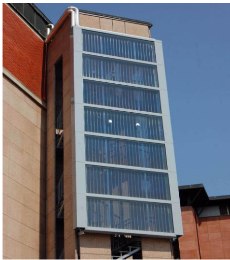
Figure 4: Prototype transparent solar thermal façade collectors, installed at the pilot building in Slovenia
