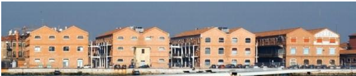
Figure 1: View of part of the warehouses
