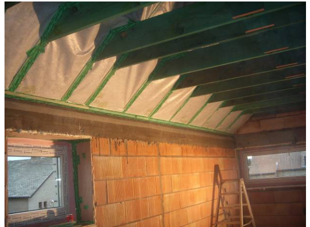
Figuur 11: Air-tight finishing of the wooden roof
