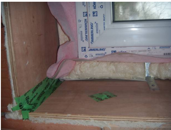
Figuur 9: Insulation and installation of the windows
