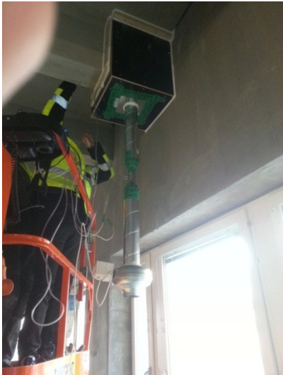
Figure 4. Equipment used for measuring air-leakages in ceiling along the outer walls
