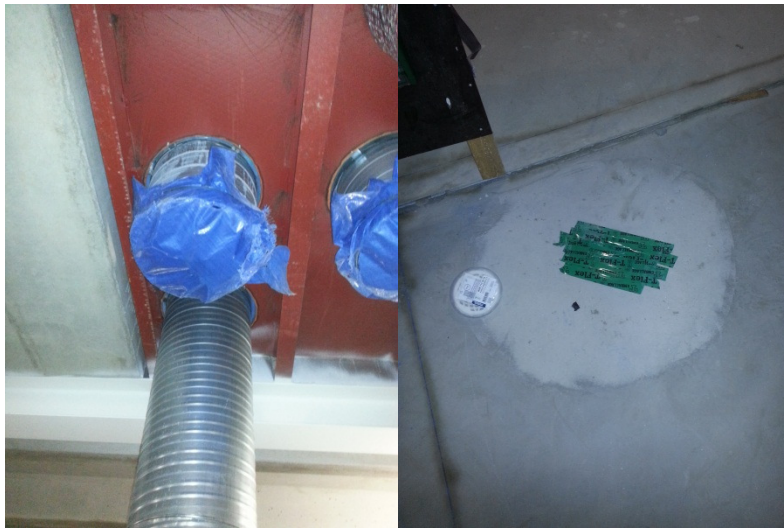
Figure 7. Temporary seals between different floors (ducts and floor drains)
