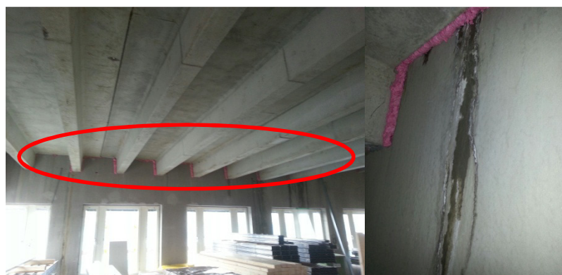
Figure 6. Ceiling along outer walls after sealing with air-tight foam
