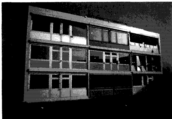
Figure 2: The LESO building, EPFL Lausanne, Switzerland
