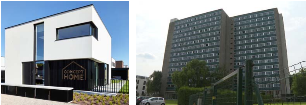
Figure 1: The single-family home (left) and the high-rise student home (right) considered in this study.
