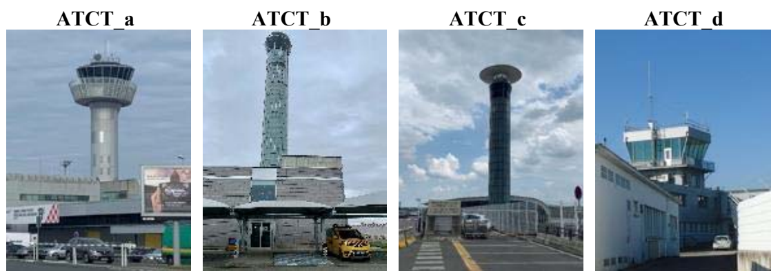
Figure 1. View of the ATCT of Bordeaux airport (a), north and south towers of Roissy airport (b and c respectively) and Grenoble airport (d)
