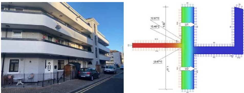
Figure 1. (a) photo of external access and external stair tower; (b) Thermal model through deck access, pre-refurb, showing ceiling temperature of 13.67C
