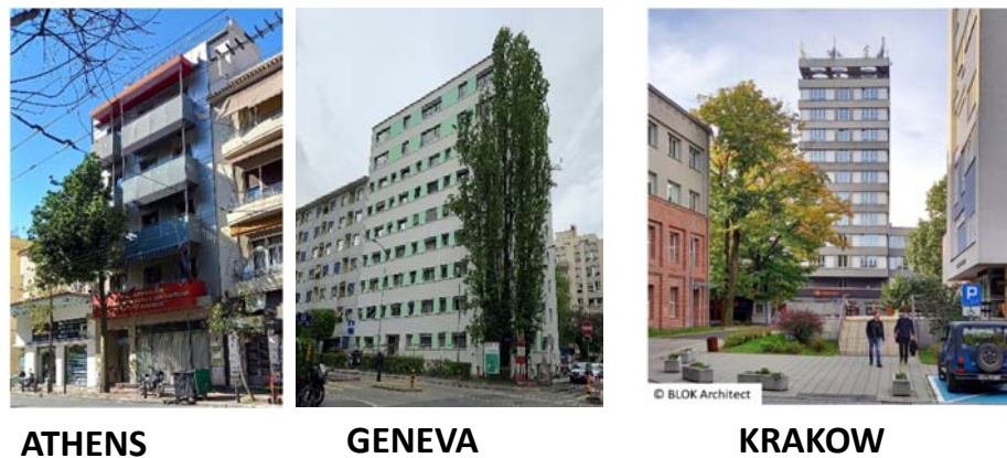
Figure 1: External view of the three test buildings
