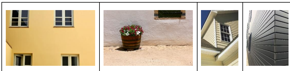
Figure 4: Examples of common exterior wall products (left to right: painted wall [29]; stucco wall [30], vinyl siding [31], metal cladding).
