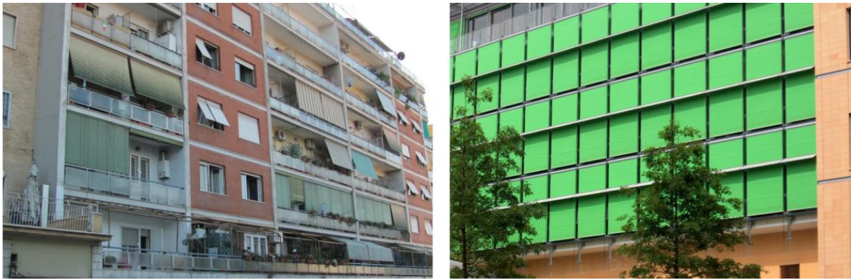
Figure 2: Individual low-cost external blinds in a social housing building in Rome, Italy (left) and the fully automated shading façade at a newspaper headquarter in Milan, Italy (right) [1].
