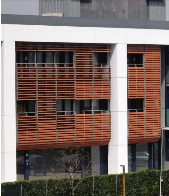
Figure 1: The wooden slats on the left figure can be tilted but not retracted. The shading system defines the façade of the building; on the right figure, fully moveable shading systems are integrated at the window level and can be operated by the users according to their requirements [1].
