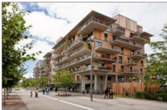
Fig.1 EXTERIOR VIEW, WEST VIEW, RESIDENTIAL PROJECT VIENNA
