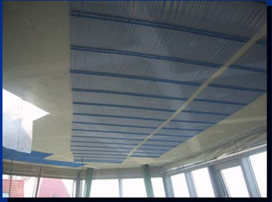
Integrated heating/cooling ceiling system with capillary mats
