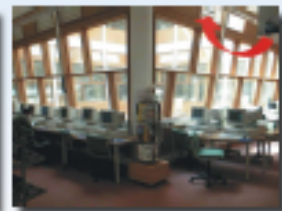
Figure 3(b) Mid-height of central light-well: air at ceiling level passes out through control louvers into the central well.
