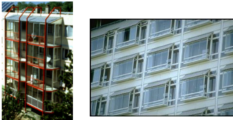
Figure 5.1. Examples of glazed balconies ( www.unl.ac.uk )
