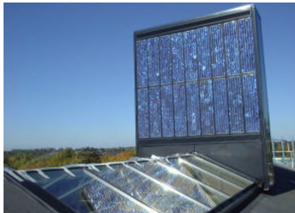
Figure 11.1 Solar Chimney at Lundebjerg, Denmark
