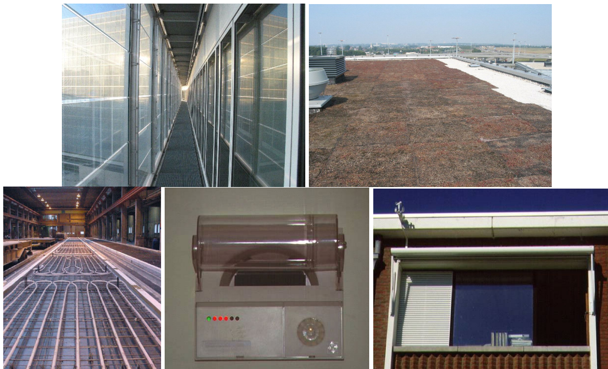
Figure 7: Examples of technologies typically not-covered by the basis calculation procedures of energy regulations a. Ventilated Double-skin Façades – b. Green roofs c. Thermal mass activation – d. Ventilation system controlled by presence detection sensor – e. Passive cooling using intensive night ventilation
