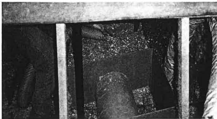
These cardboard frames are specifically designed for insulating over ducts. The walls of the boxes allow weatherizers to build up a deeper layer of insulation around long duct runs.
