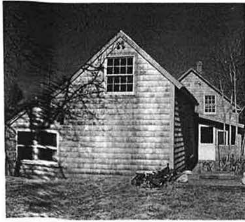
This Massachusetts farmhouse is a perfect illustration of what not to do in a remodel. The photo on the left shows the window-filled north side of the house, which is usually shaded. Previous homeowners had converted the south side (right) into an unconditioned utility room, effectively blocking solar gain for that side of the house. The current owners are looking into adding a wing with good southern exposure to bring down their heating bills.
