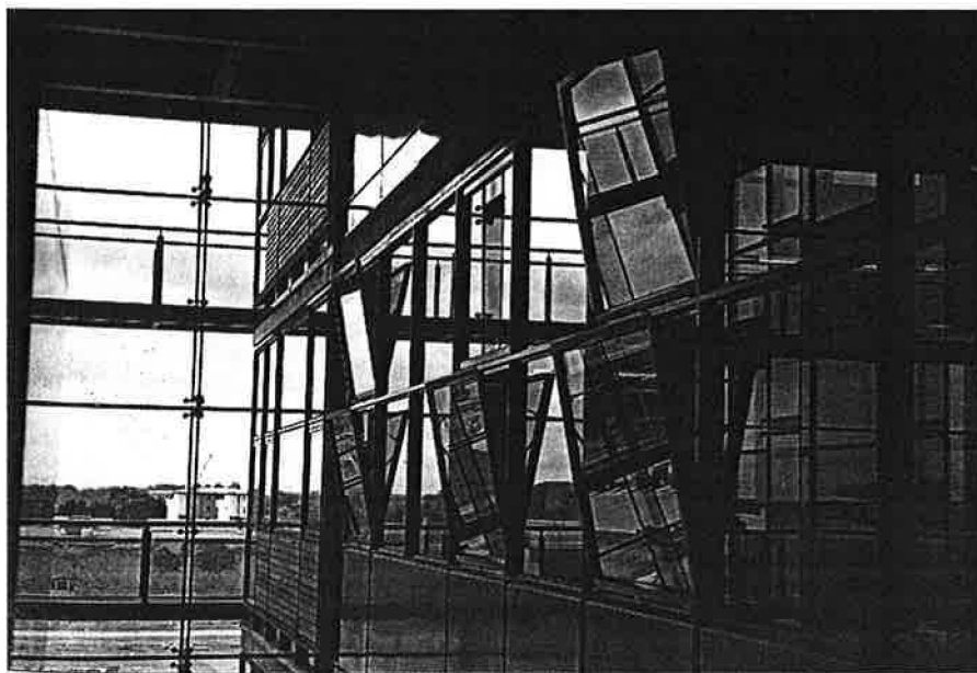
TOP: A railway line running adjacent to the University's southern elevation meant that this side of the building had to be sealed to protect it from noise ingress. However, much of the building is naturally ventilated.
