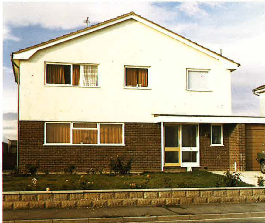
FIGURE 9 SINGLE GLAZING (UPSTAIRS) AND DOUBLE GLAZING (DOWNSTAIRS) SHOWN BY THE COOLER OUTSIDE SURFACES OF THE DOUBLE GLAZING WITH UNIFORM TEMPERATURES INSIDE. A SIMILAR IR PICTURE WOULD BE OBTAINED FOR ALL SINGLE GLAZING IF THE DOWNSTAIRS ROOMS HAD A TEMPERATURE ELEVATION ABOVE THE OUTSIDE OF ABOUT TWICE THAT OF THE UPSTAIRS ROOMS, FOR EXAMPLE, 10^{\circ}\text{C} OUTSIDE, 20^{\circ}\text{C} DOWNSTAIRS AND 15^{\circ}\text{C} UPSTAIRS.
