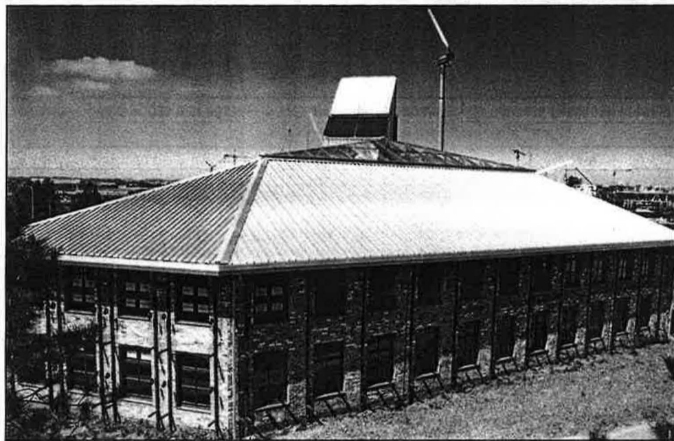
Unconventional in its appearance but conventional in its application is the Eco Centre on South Tyneside, with minimal automatic controls and a target of zero carbon-dioxide emissions.
