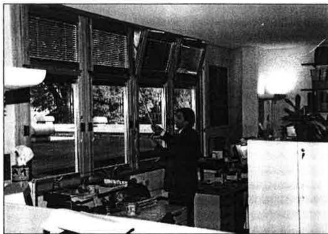
Effective control of windows and blinds helped avoid the need for air conditioning in a refurbishment of the Design Studio at the Open University, Milton Keynes.
