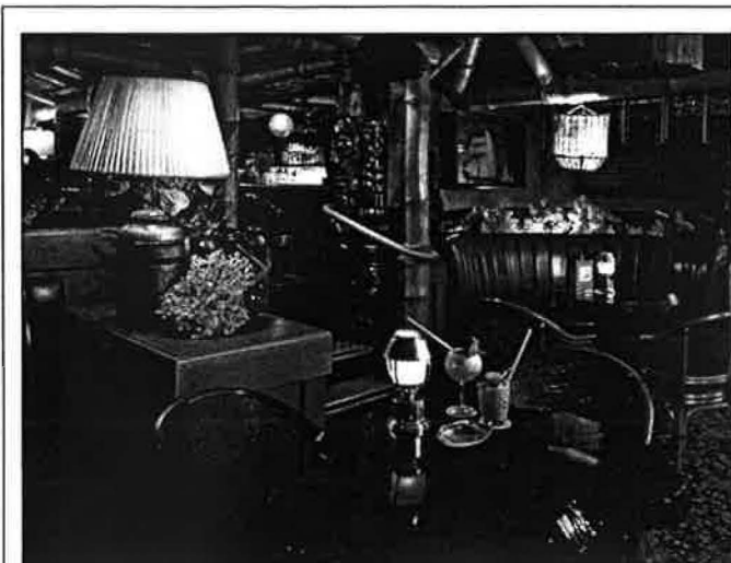
Trilon has installed an electrostatic air cleaner in Trader Vic's restaurant at the London Hilton Hotel. The unit cleans the air extracted from the restaurant and has helped improve the efficiency of the Hotel's maintenance operation, the company says. Enquiry No 210
