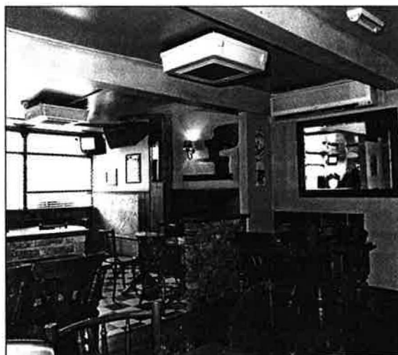
Air cleaners should be left constantly running as part of any long-term air hygiene strategy - the energy penalty is about the same as that of a domestic fridge
