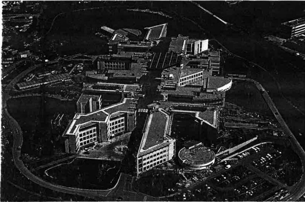
▲ Waterside comprises six, four-storey 'houses' backing on to a 175m atrium. This 'Street', with shops and bars, provides a focus for the site
